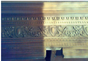
WINDOWS AND FURNITURE RESTORATION
