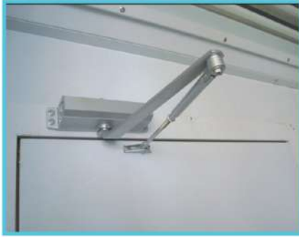
Working gate equipped with automatic position-return device
